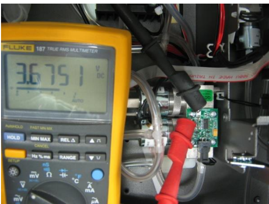
Figure 61 – Typical test point reading of manifold pressure sensor
