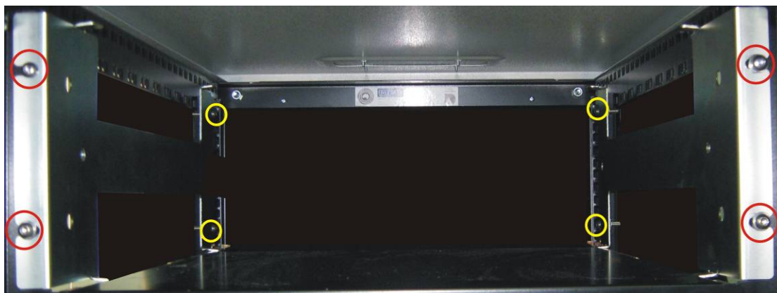
Figure 25 Installation of rack mount brackets
