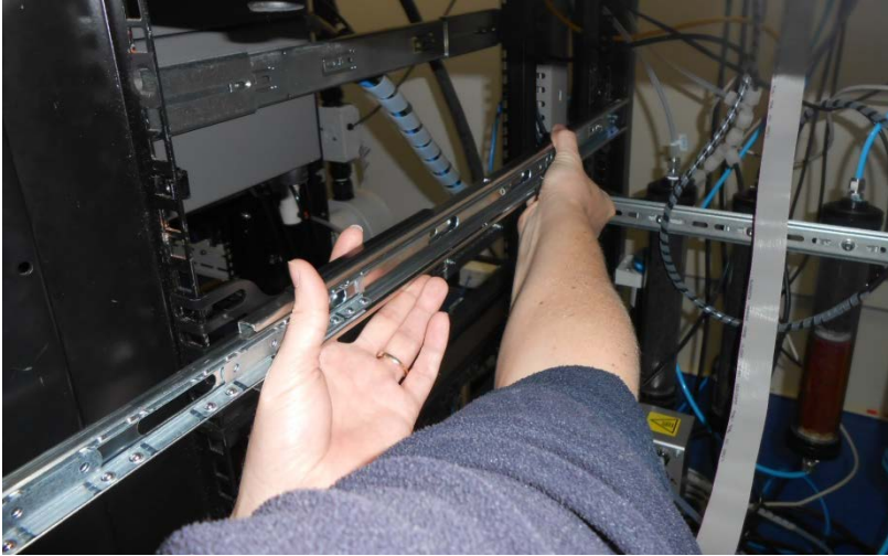
Figure 74 – Test Fit the Rack Slide Assembly into your Rack
